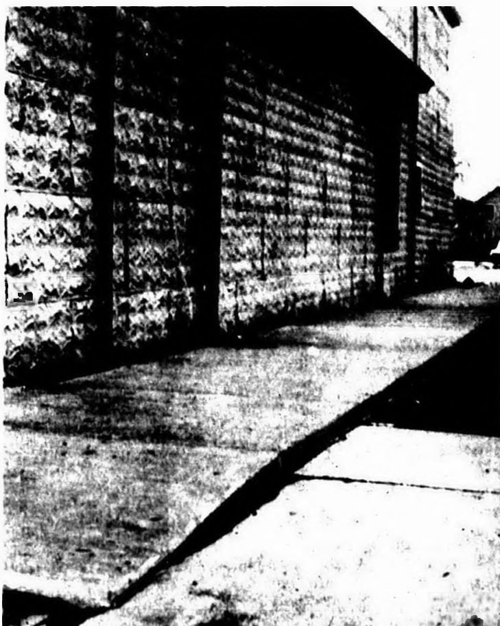
A NEW SIDEWALK was poured this week along the west side of the Grand Building. The old sidewalk was deteriorating necessitating the pouring of new cement. The sidewalk is used by the grade school children daily, to get to their respective schools. Plaindealer Photo
